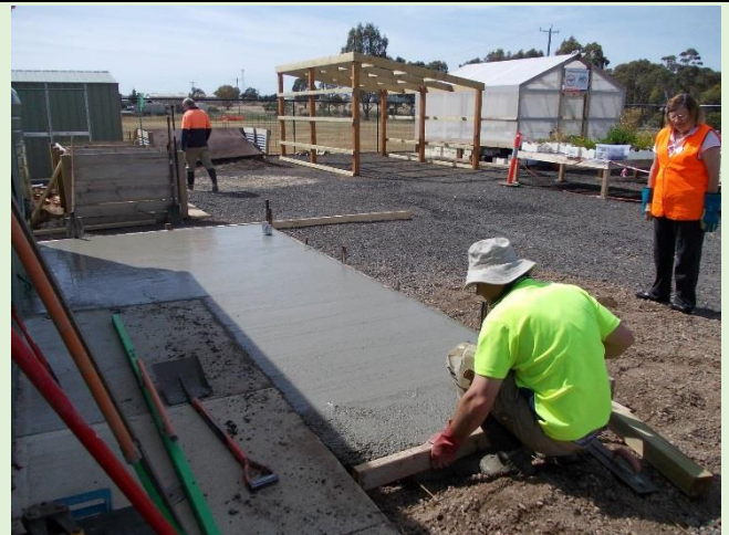
Rob the Builder laying the concrete for the wash up area
