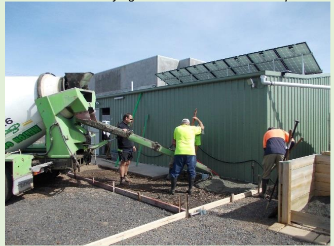
FMBG Volunteers spreading the concrete
