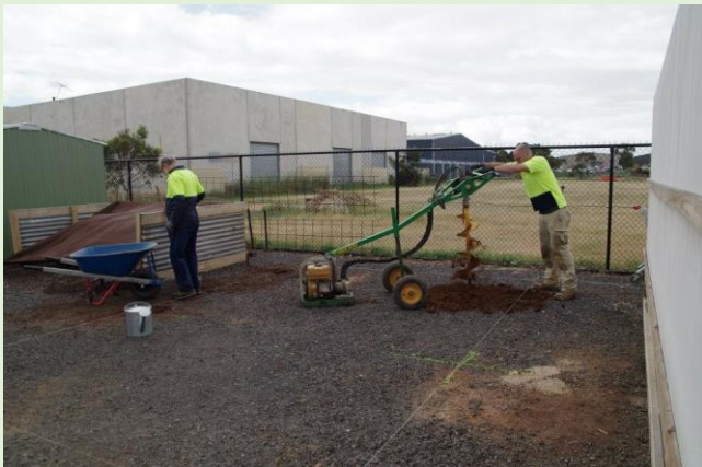
Rob the Builder drilling holes
