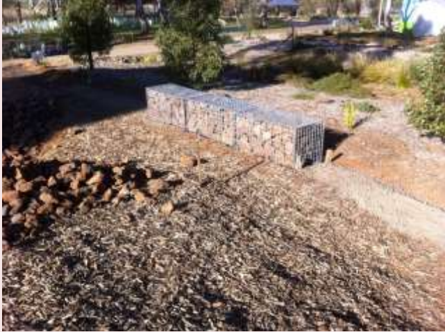
The Bushfoods Garden Gabion wall taking shape
